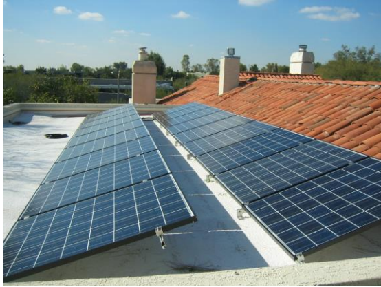
(PV panels (collectors) hidden behind a parapet wall on a flat roof)
